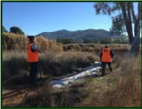
Photo: Constructing the paper, cardboard & woodchip low impact path at the Kergunyah Wetlands
